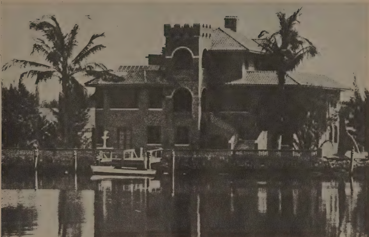
1924 — Large solar water heater at upper left on an estate at Palm Island, near Miami. From Beautiful Homes of Miami and Environs , by Kay Walker.
